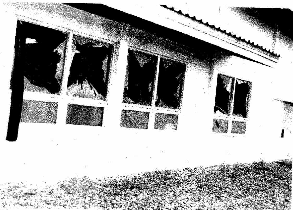
Windows of the 555th Tactical Fighter Squadron Headquarter buildings were shattered by the blast of an enemy sapper's explosive satchel charge during the Oct. 3 attack. (USAF PHOTO)
